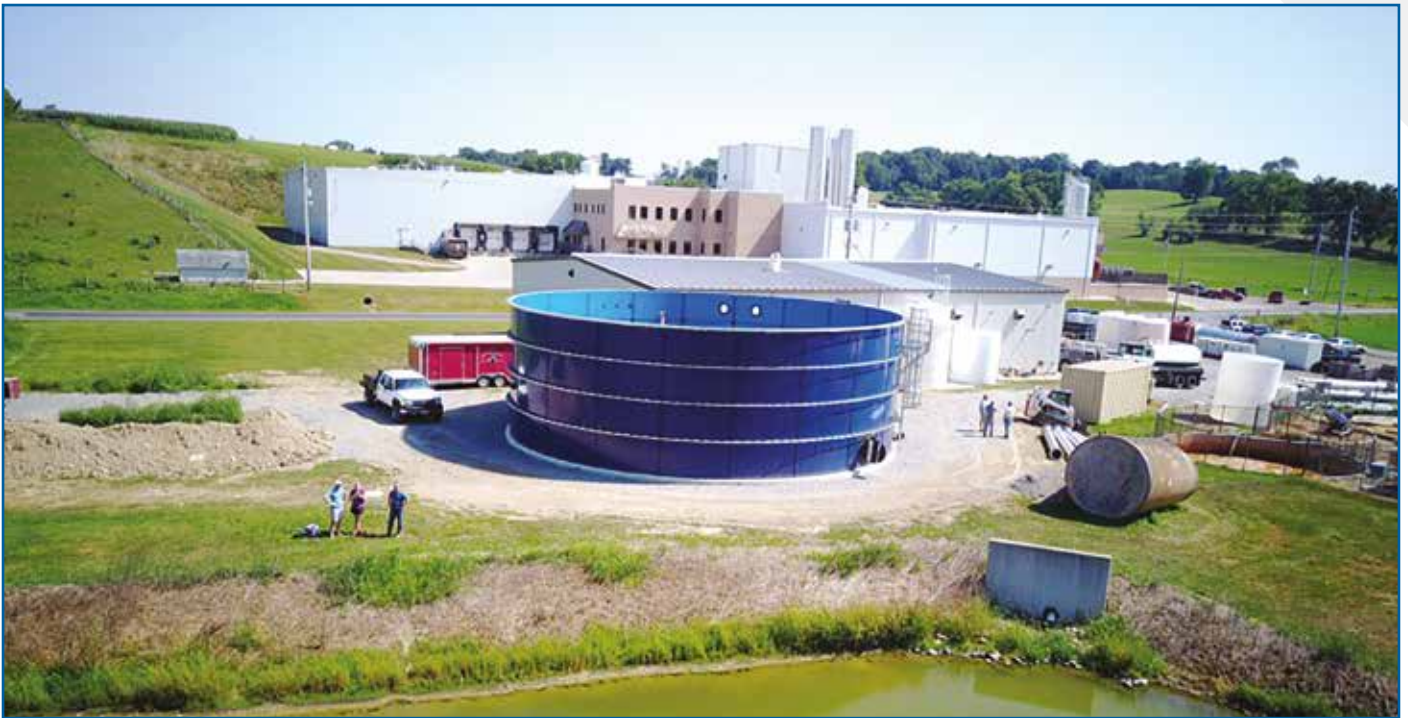
Guggisberg site with in front the bioreactor.
